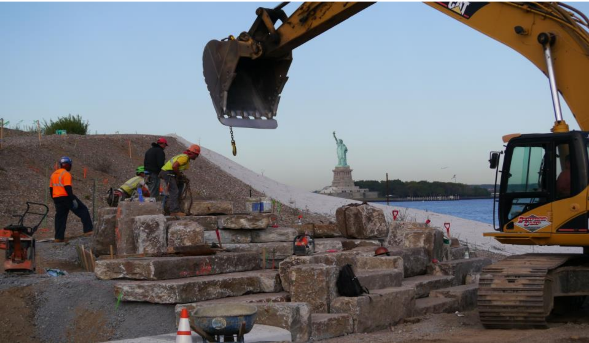
October: Installing the Granite Scramble
