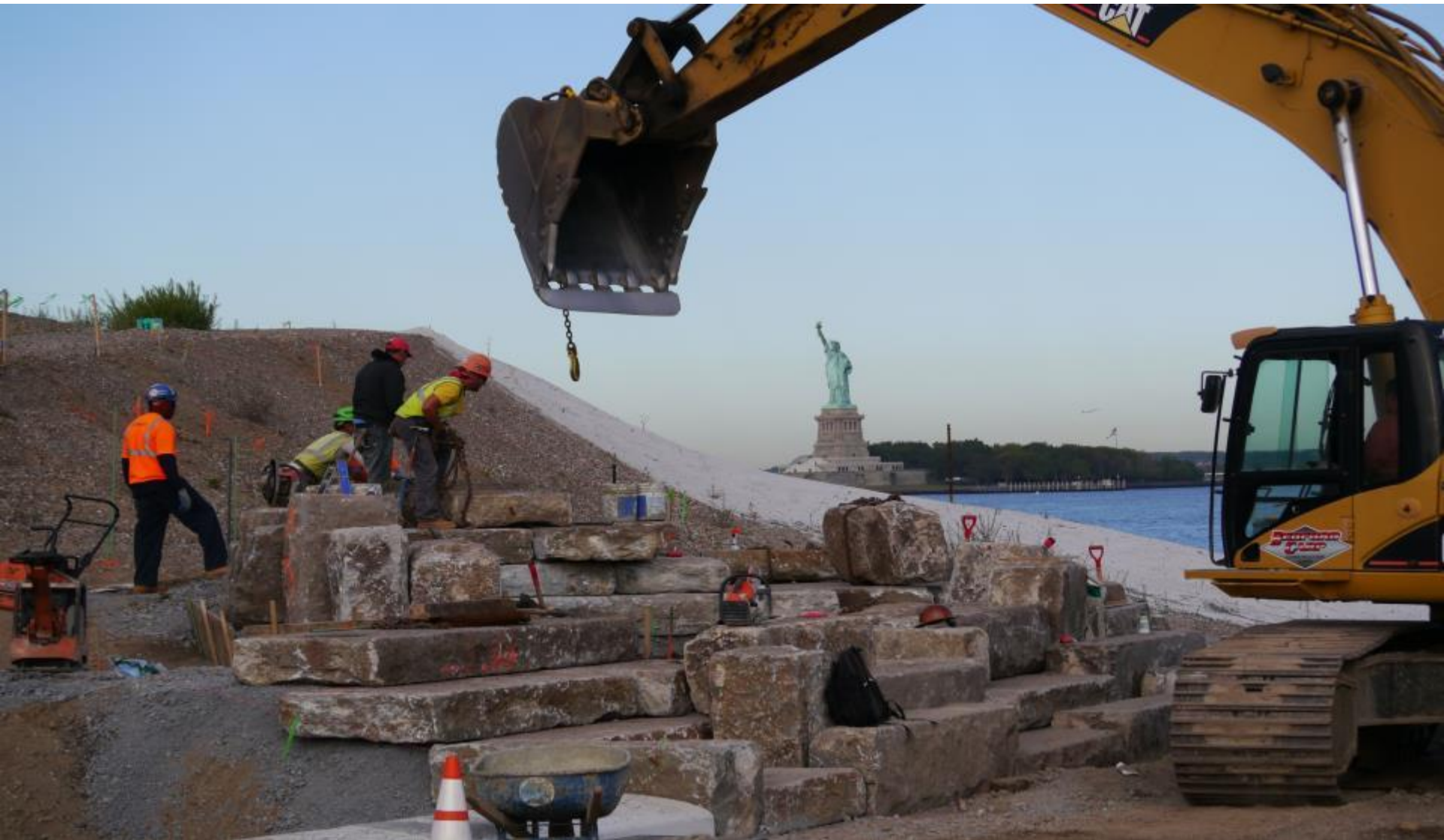
October: Installing the Granite Scramble
